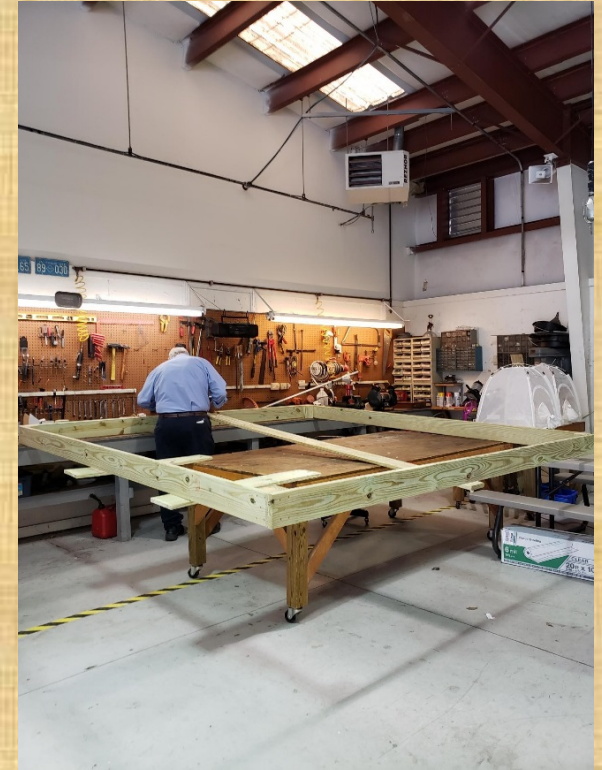
100ft bottom frame- inserting middle 1X6 for support
