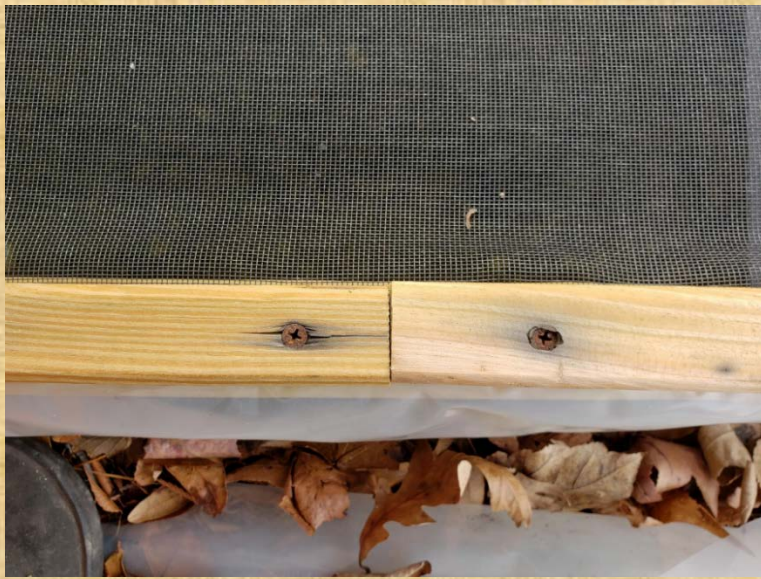
8ft 1x2 with added 2ft section to make 10ft piece. Screws were backed out one side at a time
