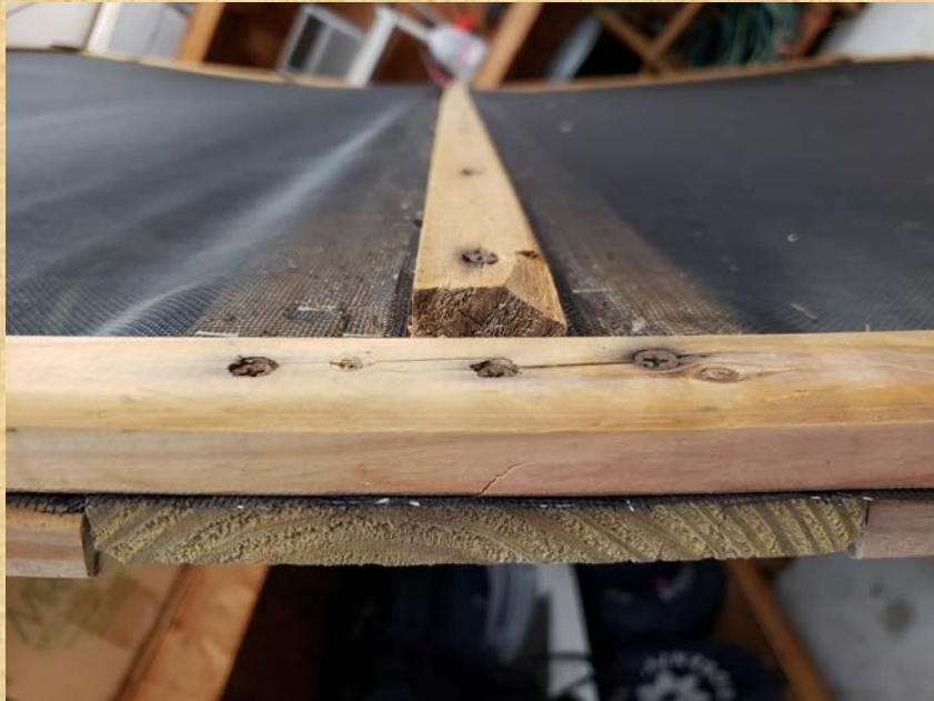
Top frame support beam (used 1x6- 10ft )
