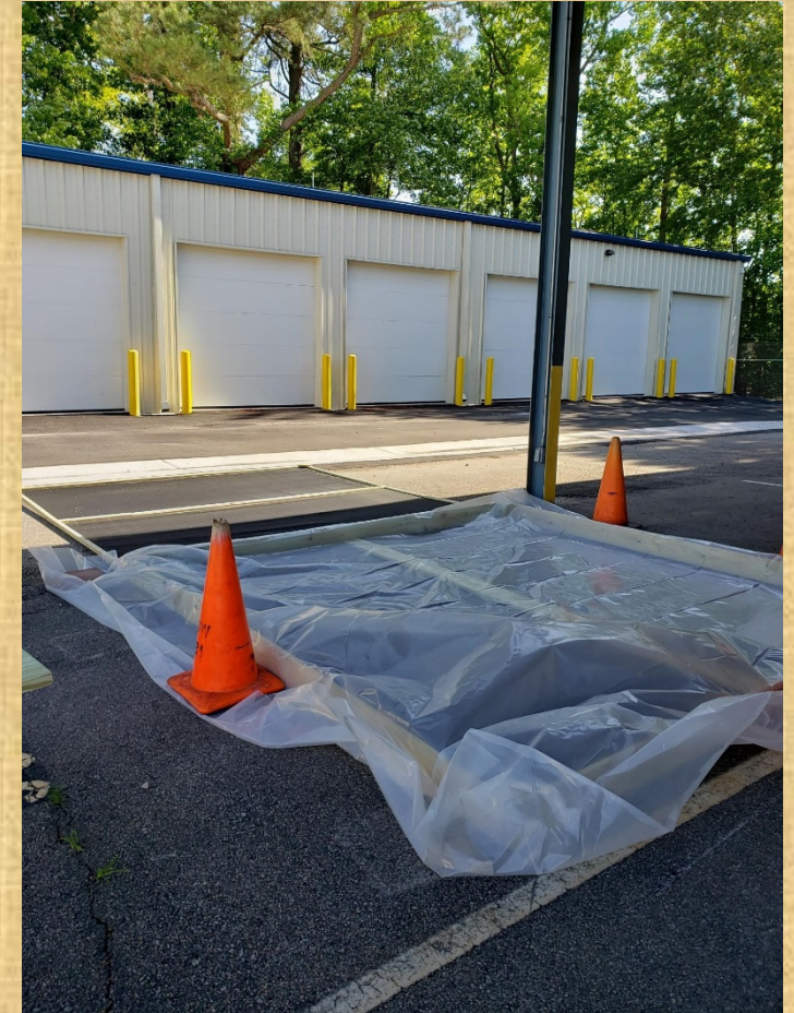
Plastic laid inside ready for water
